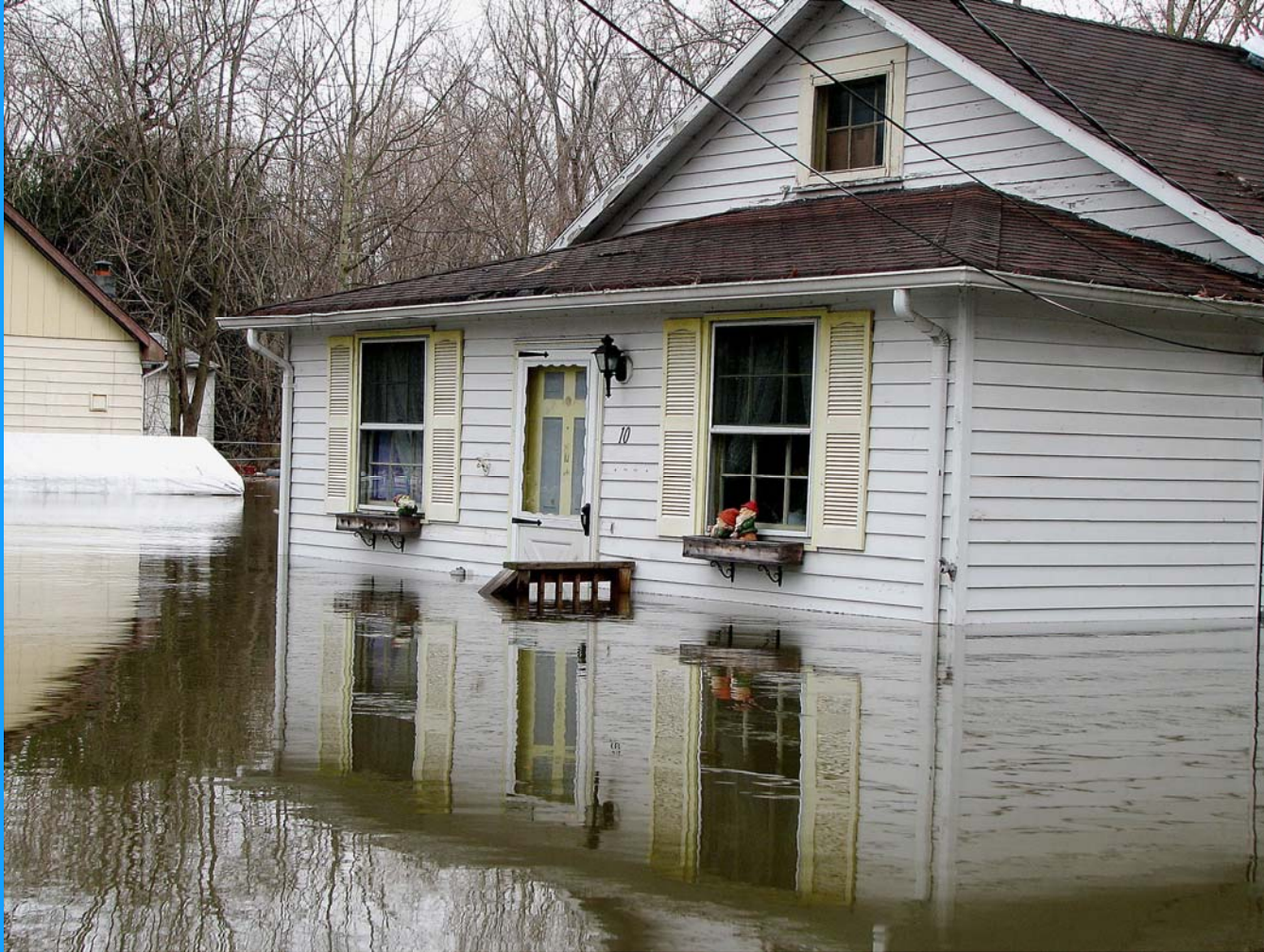
After the Flood
