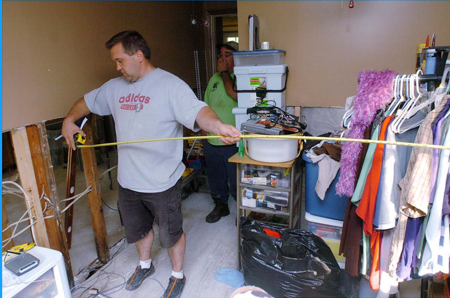
After the Flood
