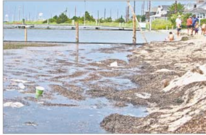
A rigid underwater fence erected to keep stingray sea nettles jellfish off the Barnegat Bay beach at Sixth Street in Seaside Park also traps dead eelgrass and litter flushed out of storm drains.
