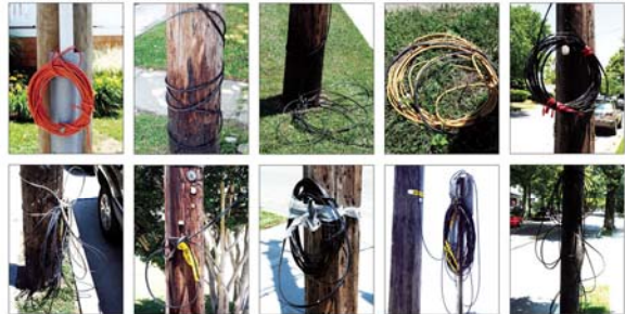
Christopher South/Cape May Star and Wave Wires storm that left the east coast left wires down all over the city - many of them were left in a hazardous manner - others wound up and taped to poles to keep them out of the streets and off the sidewalks, but still leaving the risk of wires unnecessarily left on poles by cable contractors (orange cable, top left) and you have a city-wide eyecore that was not being addressed until pointed out to utility companies by the Star and Wave.
