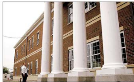
Borough Administrator Greg Franz inspects the newly completed borough hall building, which the town could begin moving to by mid-September.
