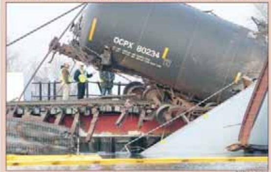
Workers investigate how the train derailed after the bridge collapsed in Paulsboro Friday morning after the bridge derailed by several cars fell. At least one car was carrying the chemical vinyl chloride.
