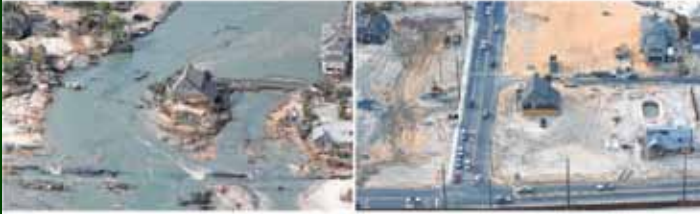
In Monmouth, Sandy created a tidal barrier between ocean and bay with a house in the middle. Today, right, the beach is closed and the house is again surrounded by water.
