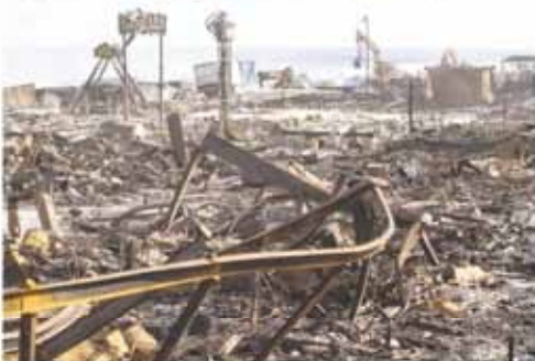
Debris at Seaside beach along the boardwalk and Seaside Heights boardwalk is seen looking south from the upper deck of the Boardwalk Hotel at what remains of the Park Plaza. The structure was destroyed.
