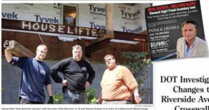
House After Paper Scaffolding Installed with its owner, Peter Novotny, Jr. It and Sharon Novotny sit in front of a 4,000-sq-ft "Ranch House".
