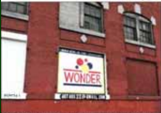
OLD BREAD, NEW BREAD – The complex of buildings occupying nearly a city block between Clinton and Grand, Seventh and Eighth streets, is about to make way for new residential buildings.
