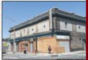
THE NEW KINGS CROSSING, a new development on King Drive.
