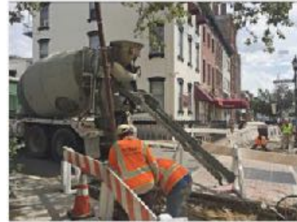
Construction on Washington Street won't be completed until July 2018.
