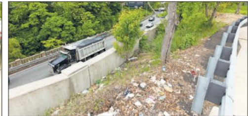
IT'S A short distance in spots between the sidewalk and the exposed portions of the lower roadway along Route 139 between Kennedy Boulevard and Collard Street in Jersey City.
