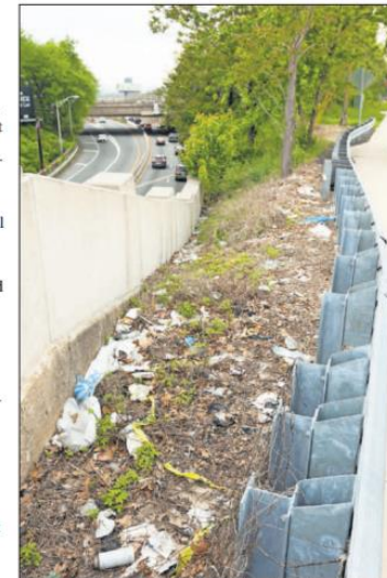
TRASH LITTERS the area between the sidewalk and the lower roadway wall along Route 139 between Kennedy Boulevard and Collard Street in Jersey City.
