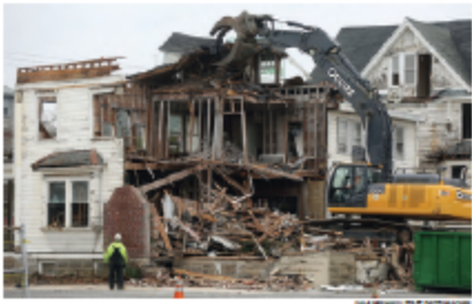
Photograph of a large building being demolished.
