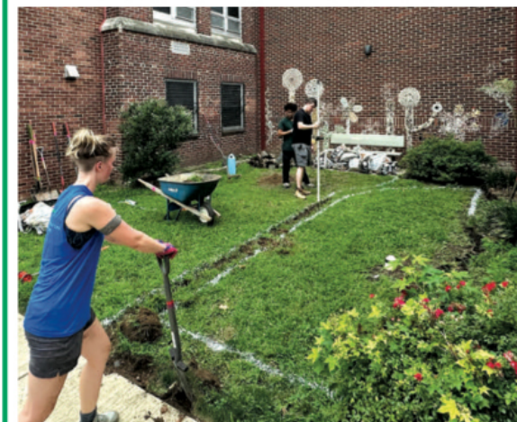
A GARDEN GROWS: A lush new rain garden was installed at Edison elementary school in Haddon Township this week. The garden is the product of a grant administered by the Rutgers Cooperative Extension and under their water resources program. The project was a joint effort between local organizations and the university to collect and filter stormwater.
