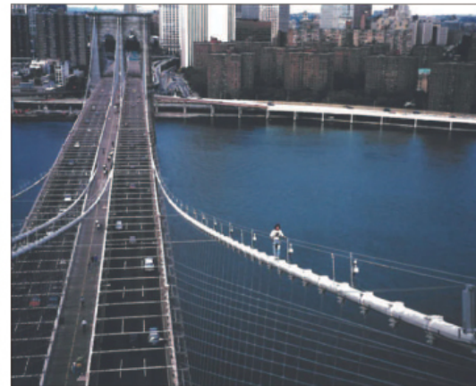
In 1997, bridge enthusiast Bill Campbell, a Court House resident, convinced New York City to give him a permit to climb to the top of the Brooklyn Bridge.
